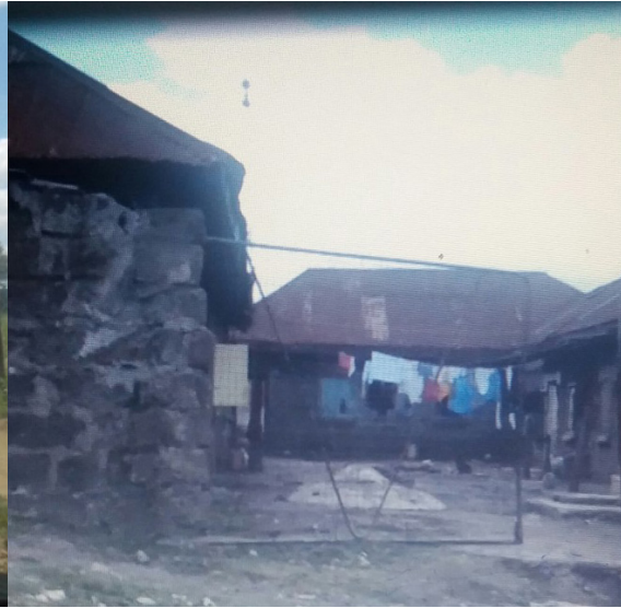
Private dilapidated residential houses in the older part of town within the planning area
