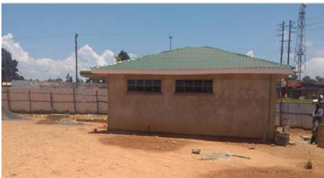
Figure 5: Ablution block in Sabatia Bus Park under construction
