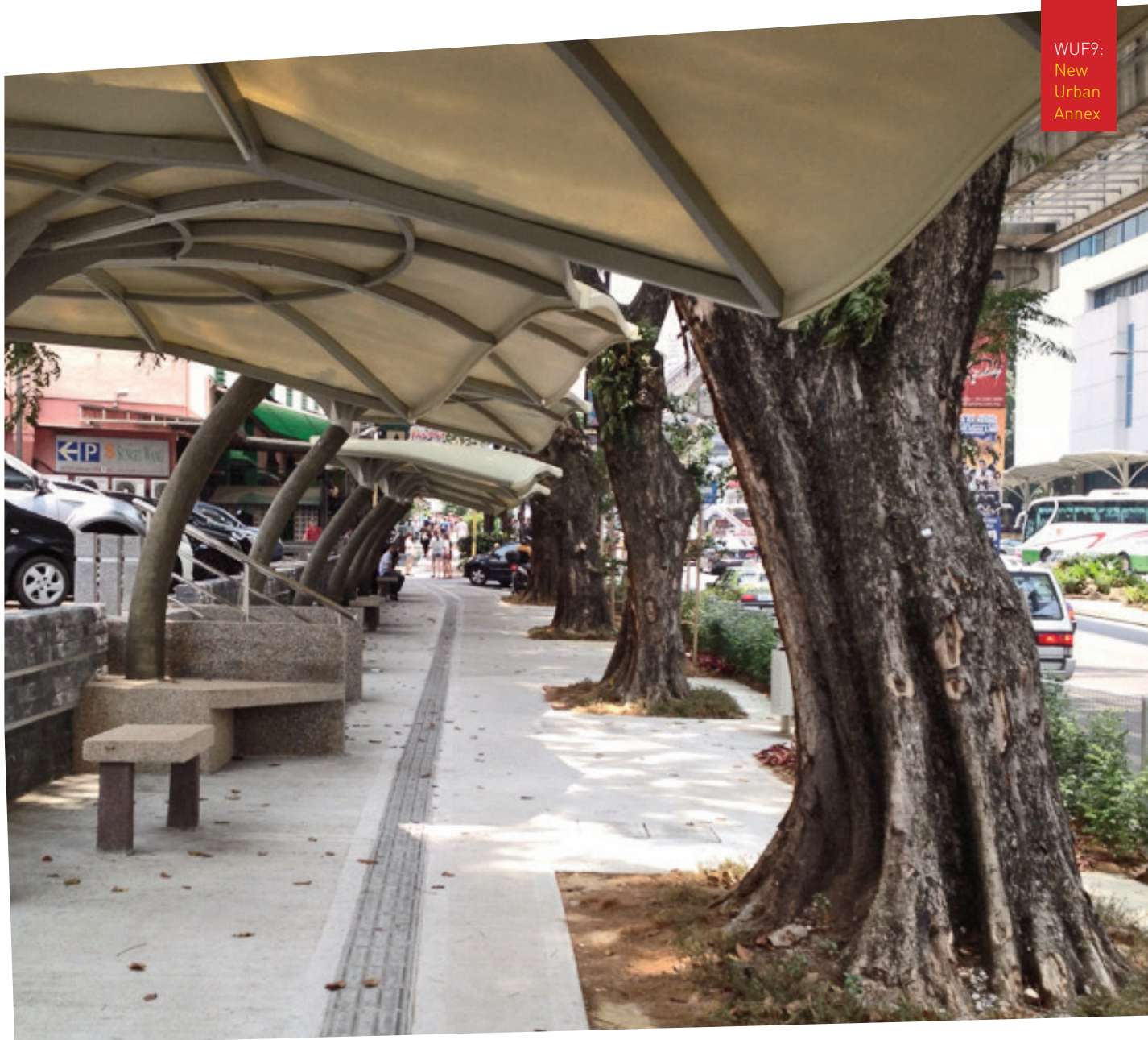
A sheltered walkway in Kuala Lumpur, Malaysia.
