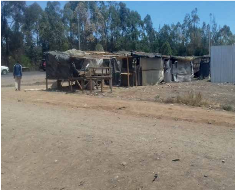
Temporary structures/shed along the A2 highway
