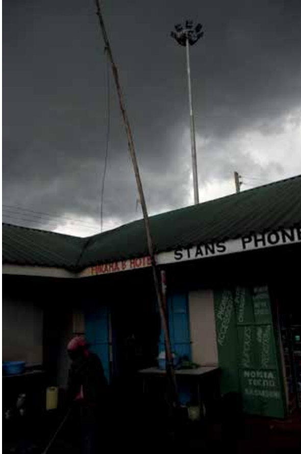
Erecting high-mast floodlights has positively contributed to the local economy.
